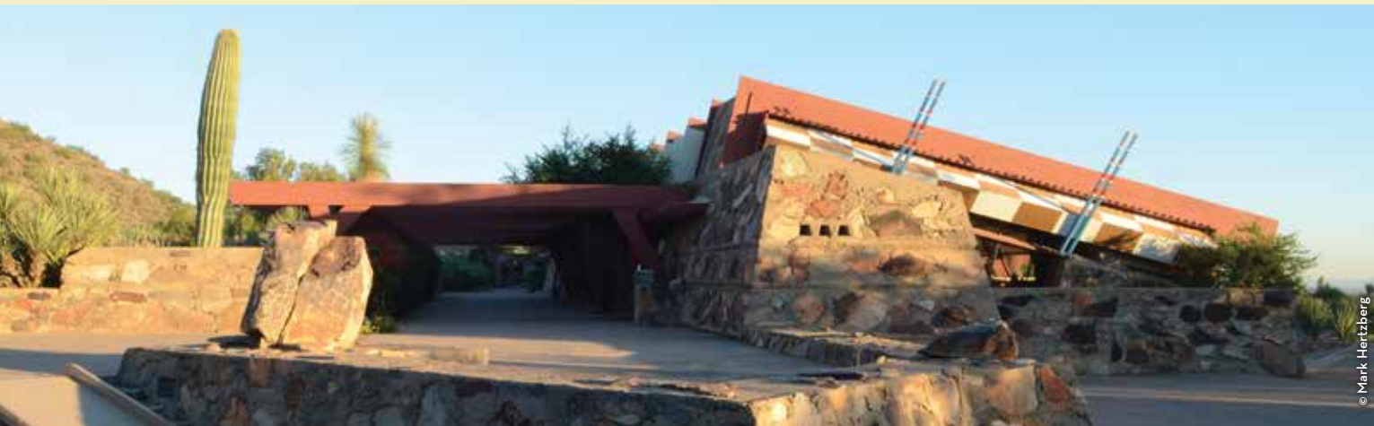
The pergola and drafting room in the setting sun at Taliesin West in Scottsdale, Ariz.
